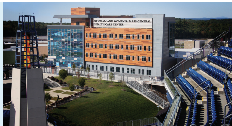
Brigham and Women's/Mass General Health Care Center at Patriot Place is a modern, four-story building adjacent to the entrance of Gillette Stadium.
